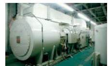
Flywheel-type train line power storage equipment
