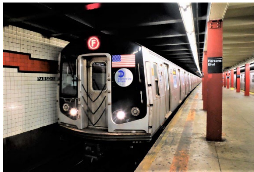
Queens Boulevard Line
